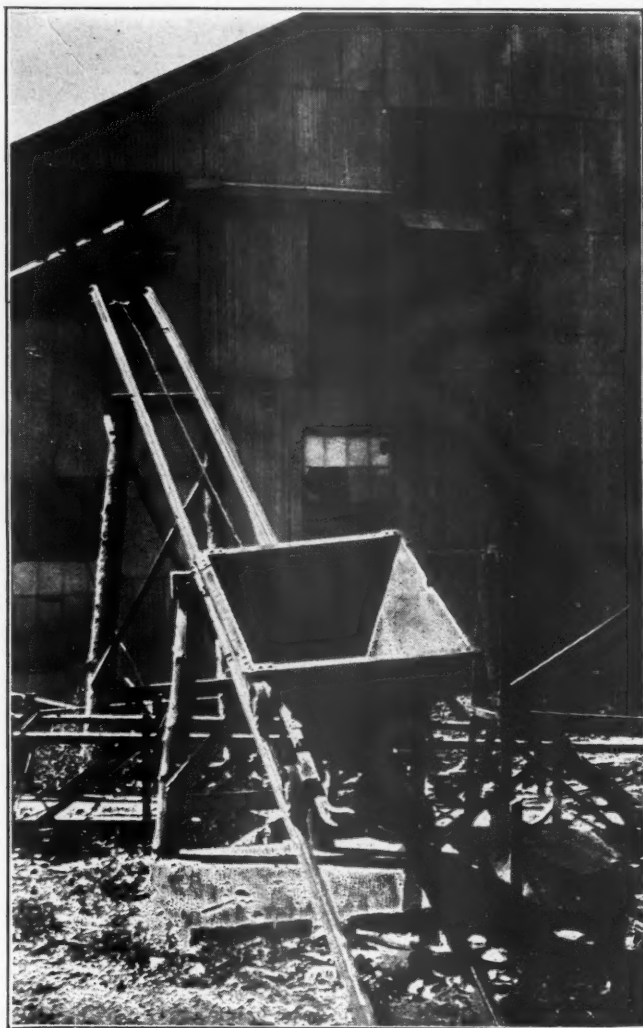
Incline for Bringing Coal from Storage Hopper to Firing Floor
